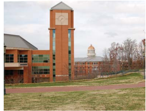
Photos courtesy of Turner Construction Company
